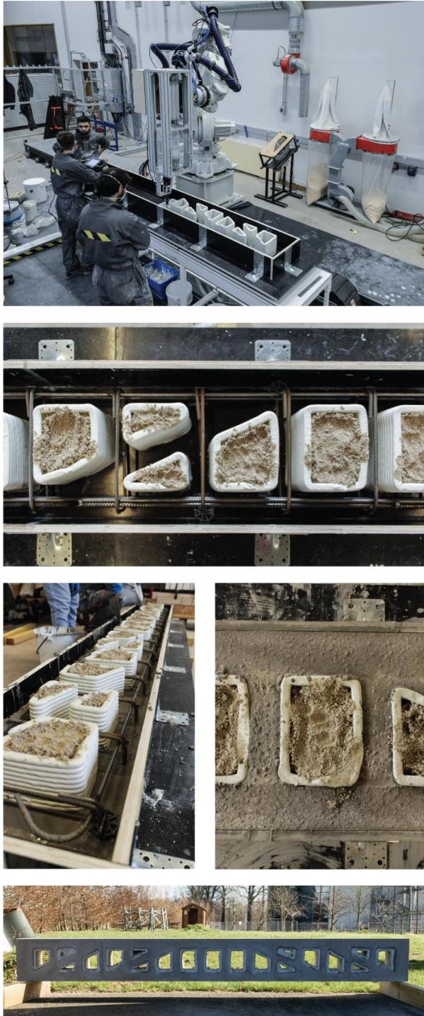
Figure 6. Fabrication of the second prototype. From top to bottom: printing of the moulds, insertion of the rebars and filling of the moulds with sand, pouring of the concrete, demoulded beam.
